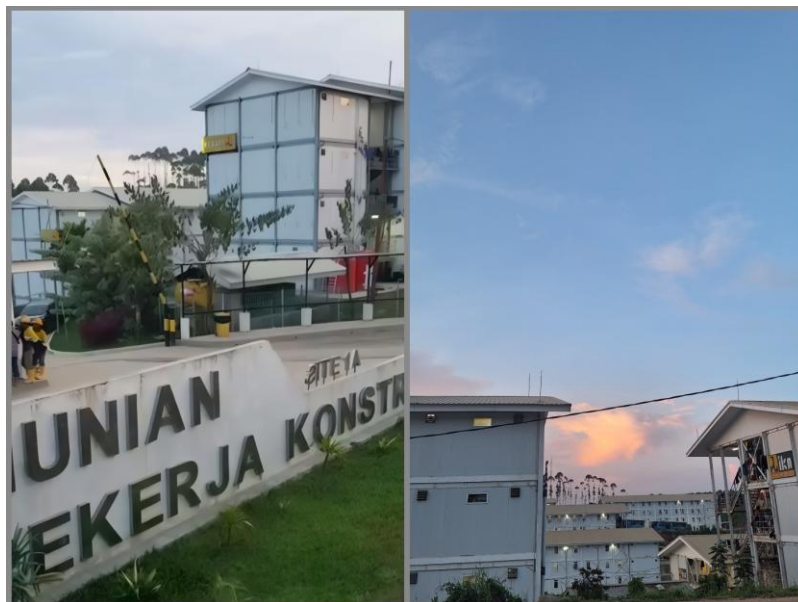
Figure 2. Construction Worker Housing (HPK) Source: Author's Documentation (2024)
