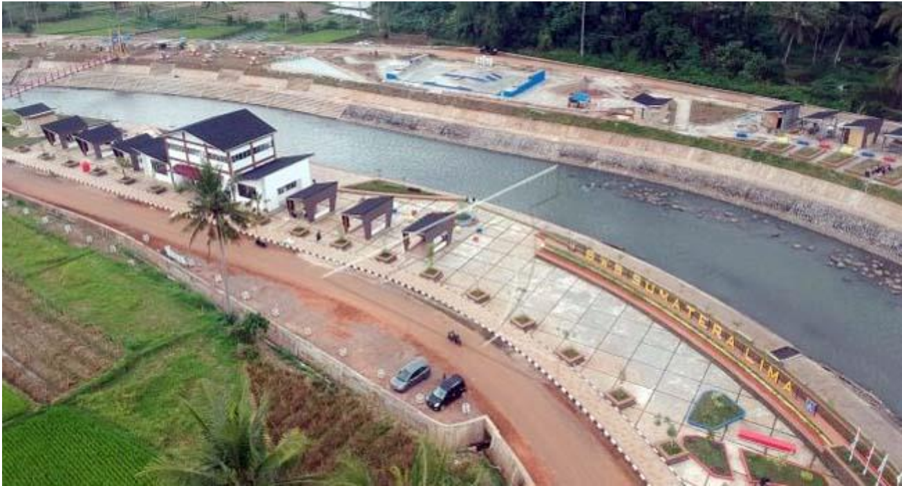
Figure 7. The condition of the Batang Agam River bank after normalization Source: https://hariansinggalang.co.id/ada-basianyuk-dan-barakik-pada-festival-batang-agam/
